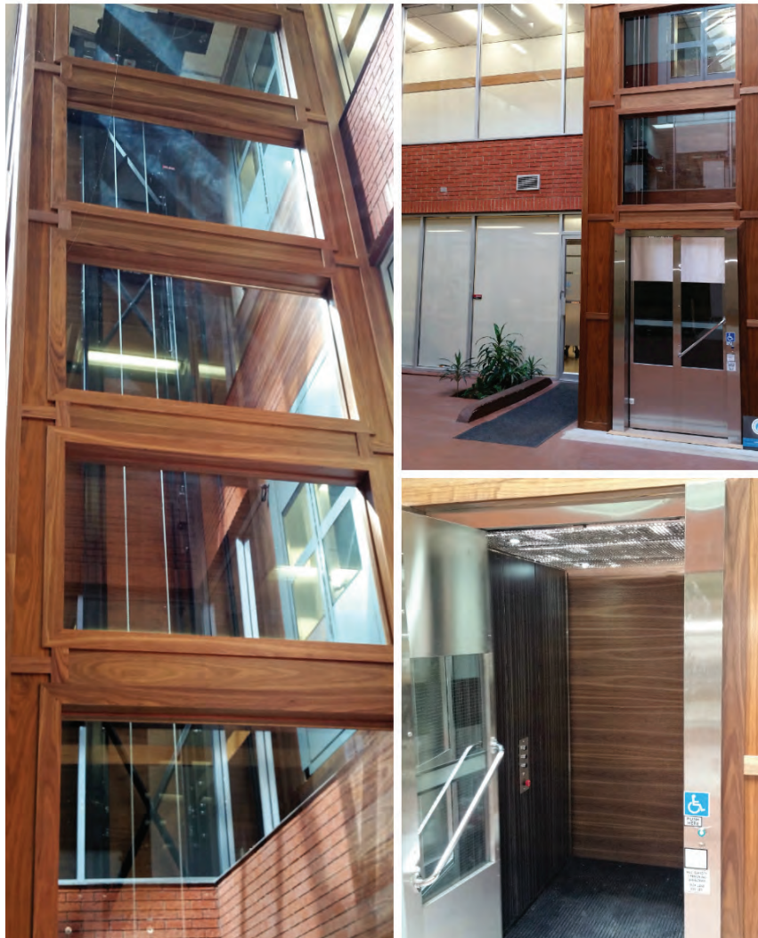
Figure 1: A full-height-carriage lift; photos courtesy of Uppercut Elevators and Lifts
