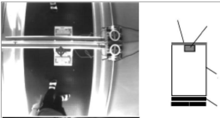
Figure 4: Incorrect mounting location for ESPROS/VOL-V in ceiling of elevator cab near mirrored back wall
